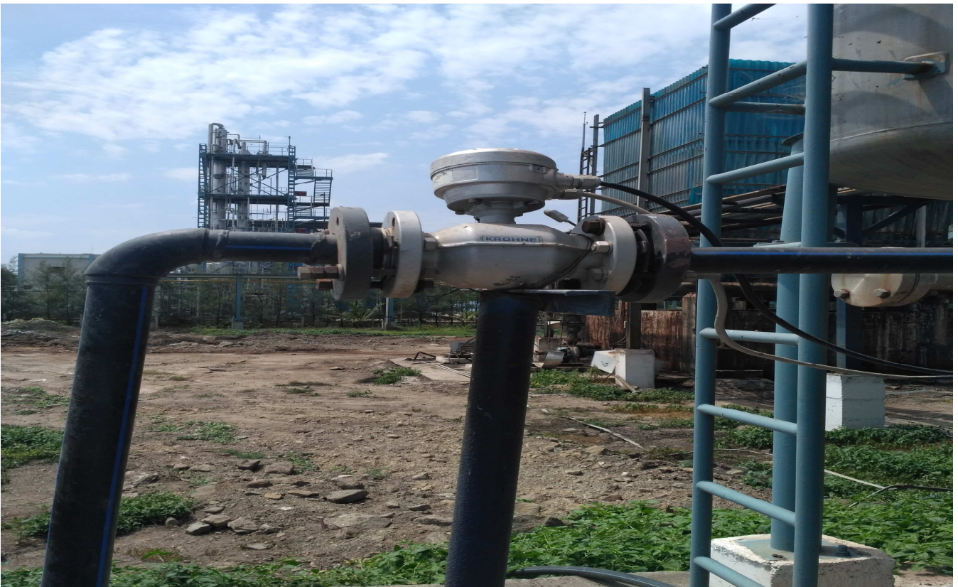
Image 2 : Magnetic Flow Meter
