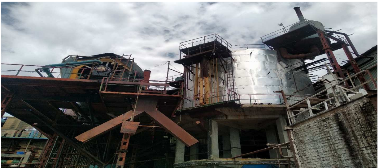
Clarifier & Vacuum filter one no. added
