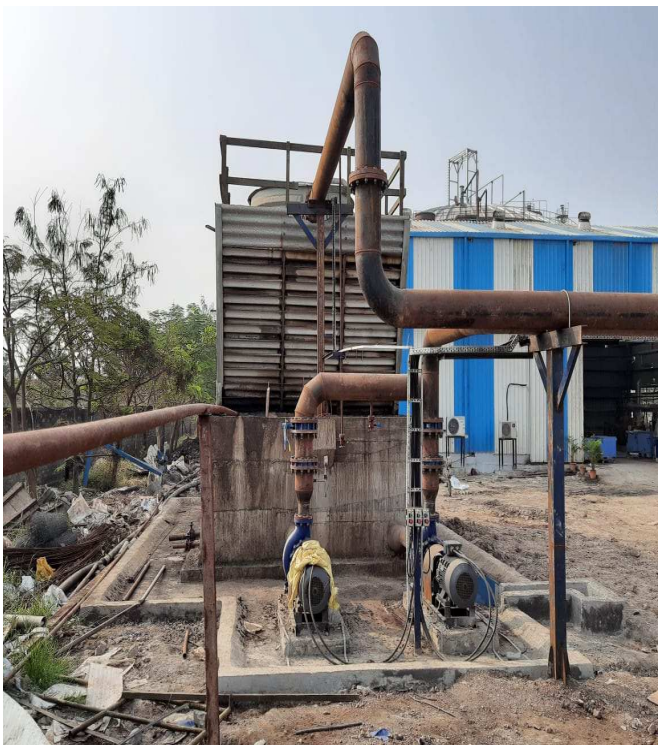
Cooling Tower installation
