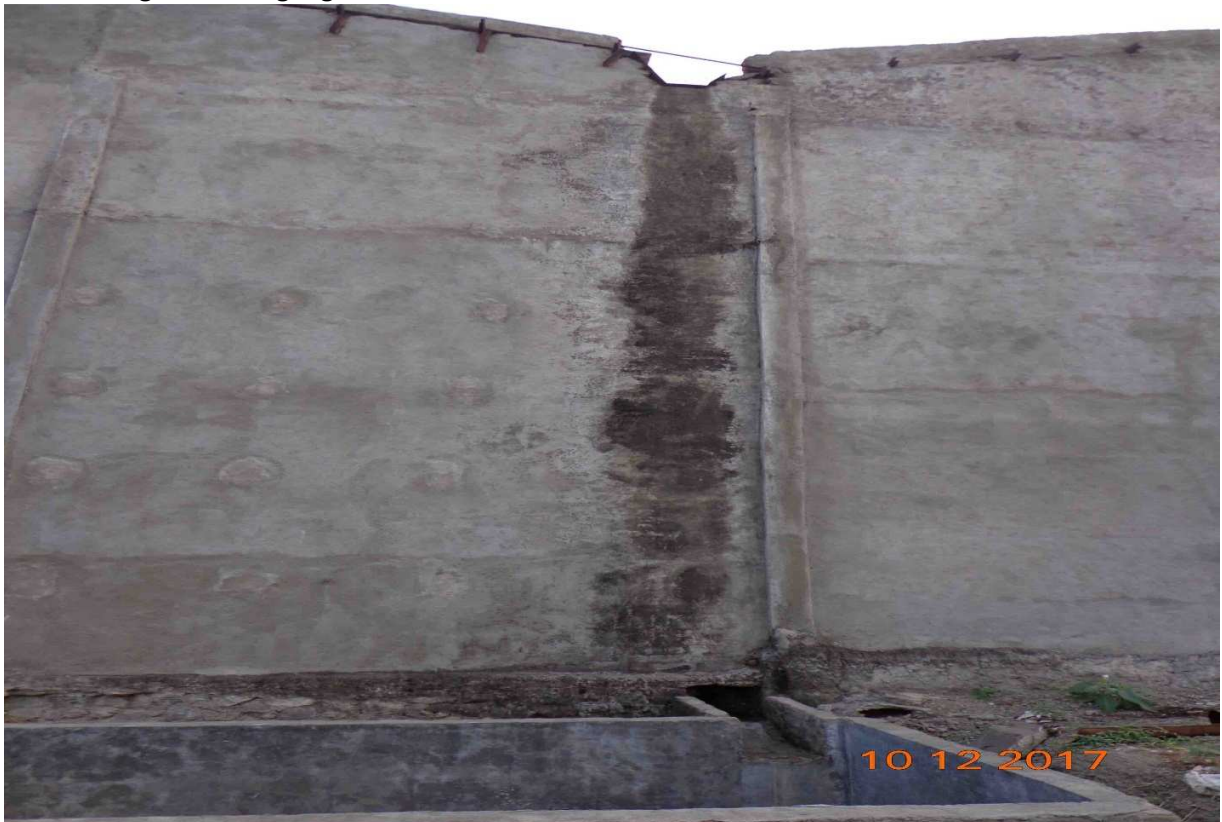
Rain water gutter of sugar godown
