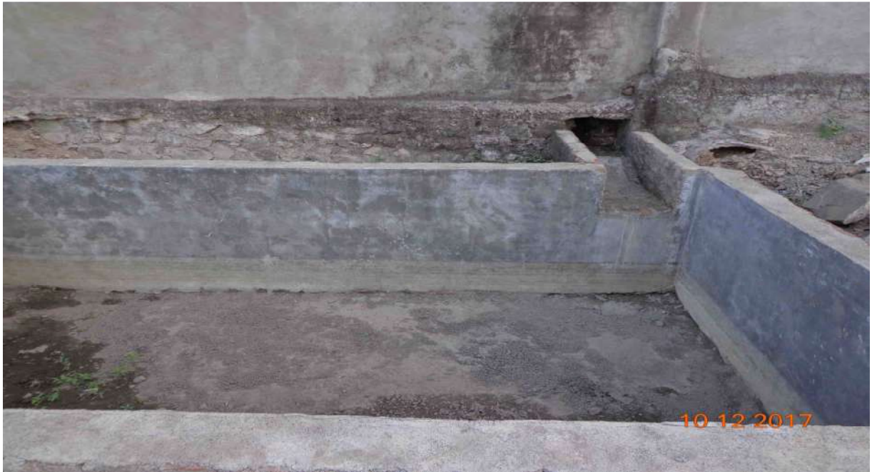
Rain water Near sugar godown collection tank
