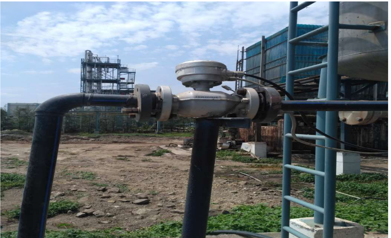
Image 2 : Magnetic Flow Meter
