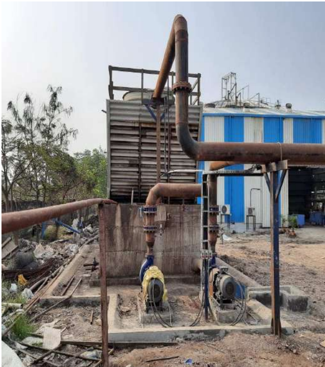
Cooling Tower installation
