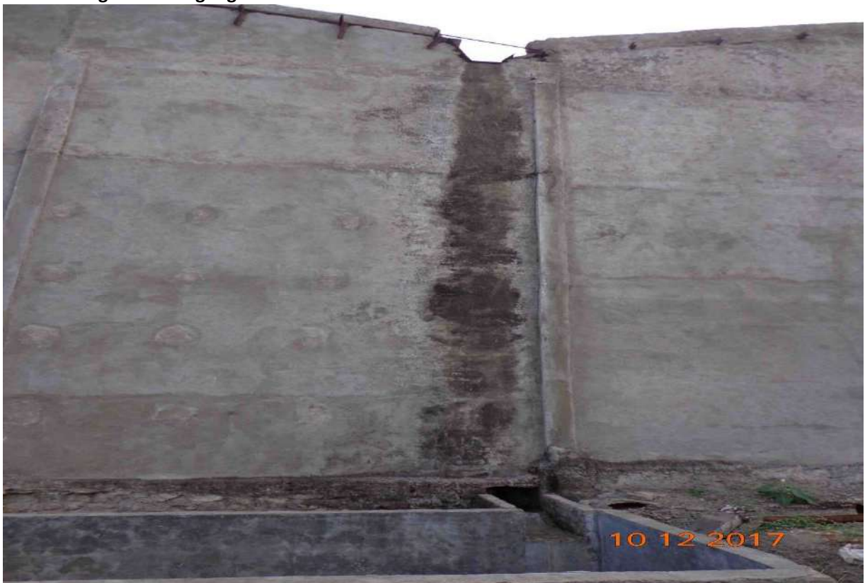
Rain water gutter of sugar godown
