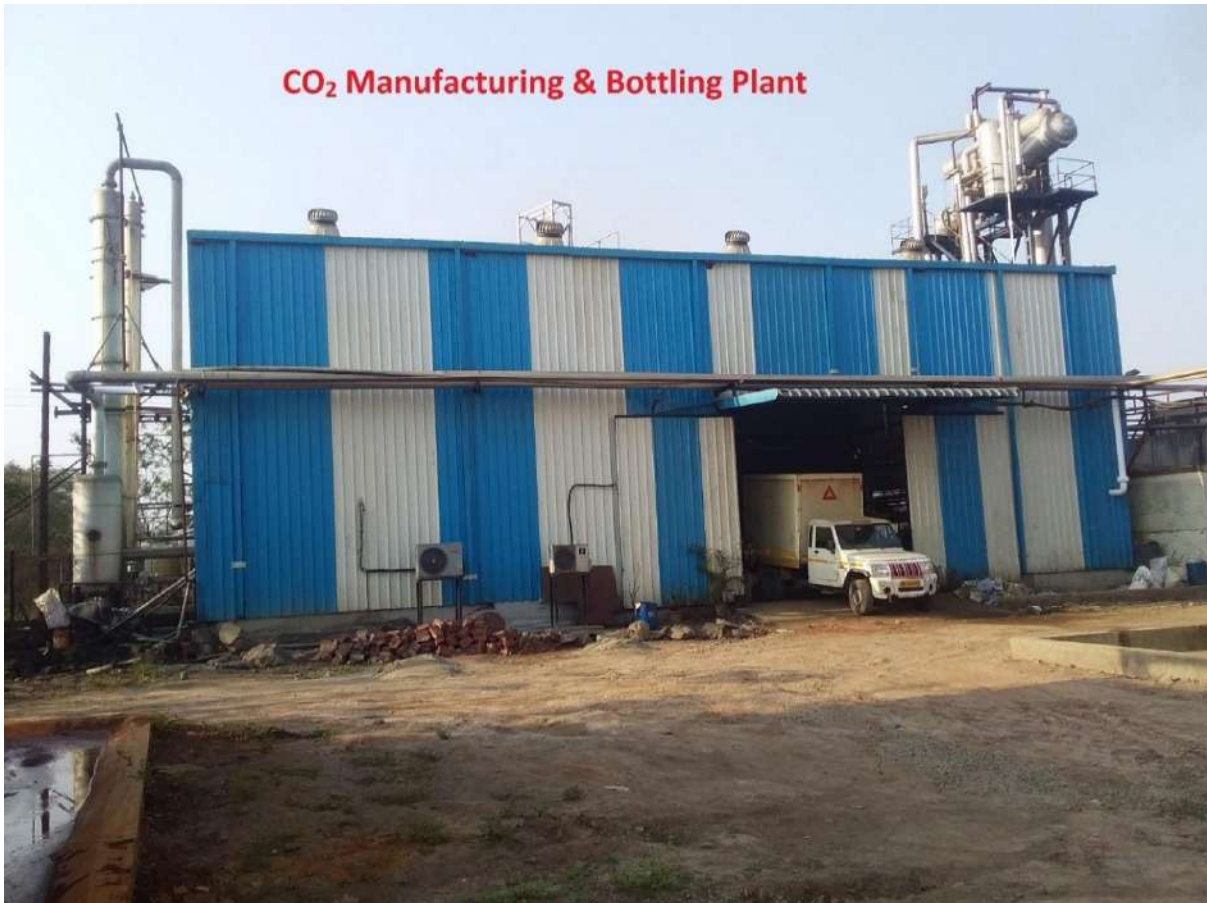
CO 2 Manufacturing (Liquid CO 2 & Dry ice) Plant-Shreenath Mhaskoba Sakhar Karkhana Ltd.
